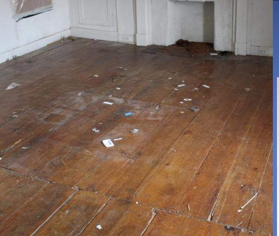
Seam in flooring and baseboard molding indicates extension to the West
